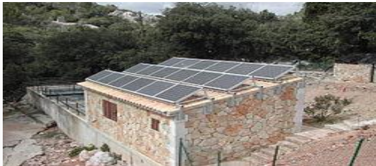
A sewage treatment plant that uses solar energy
